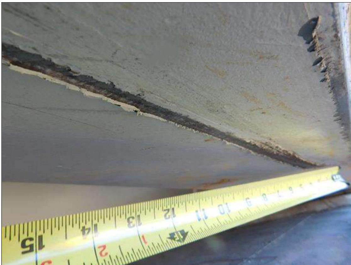
Span 1 Beam 1: IMPACT DAMAGE - THERE IS A 1'-8" LONG X 1/2" WIDE X 1/16" DEEP SCRAP ON THE BOTTOM FLANGE AT 12' OUT FROM END BENT 1 .
