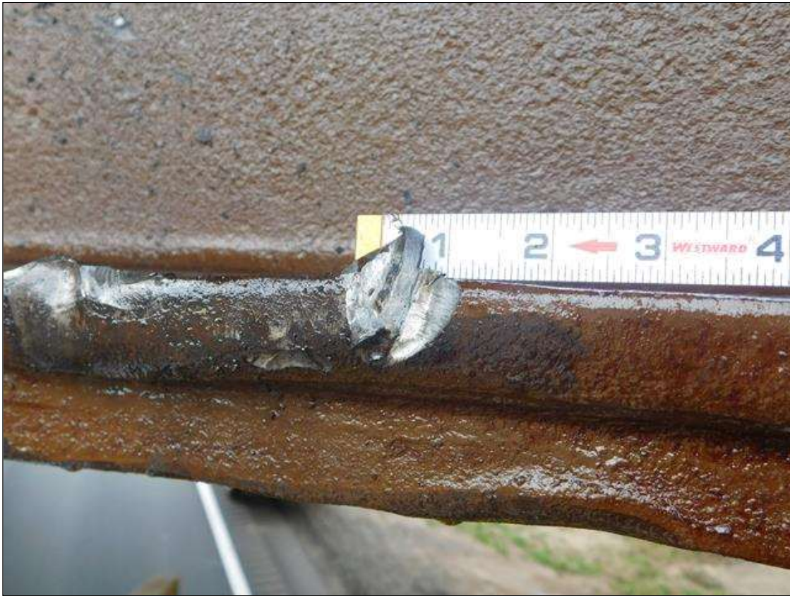
Span 3 : INDENTATION IN BEAM 6 STARTING AT 44' 4" FROM INTERIOR BENT 3. 1" LONG BY 1/4" DEEP
