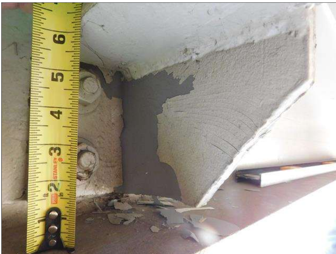
IMPACT DAMAGE - DIAPHRAGM 1 BAY 1 LEFT SIDE THE LOWER 8" OF DIAPHRAGM DEFLECTED NORTHWARD UP TO 2"
