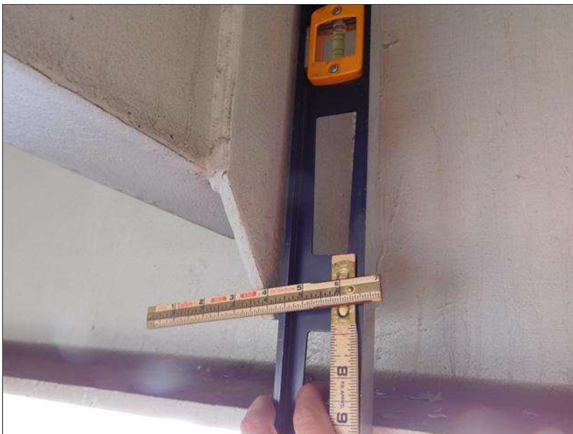
DIAPHRAGM 4 BAY 9 IS OUT OF PLUMB SOUTHWARD FOR 3/4"
