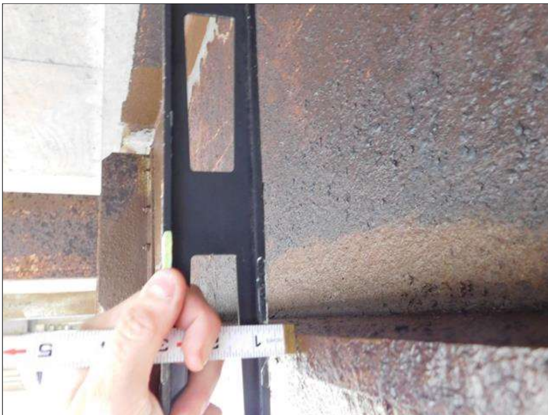
Span 3 : BEAM 5 SWEEP EASTWARD 1" FOR A LENGTH OF 5' AT 47' -10" OUT FROM IB 3. CONFIRMED BY SPECIAL INSPECTION ON 3/5/19.
