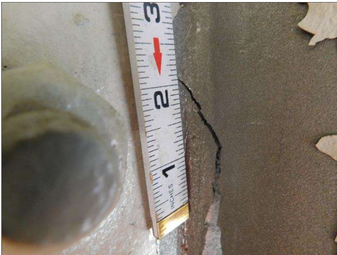
2" LONG CRACK IN TOP OF RIP IN DIAPGRAGM 2 BAY 2
