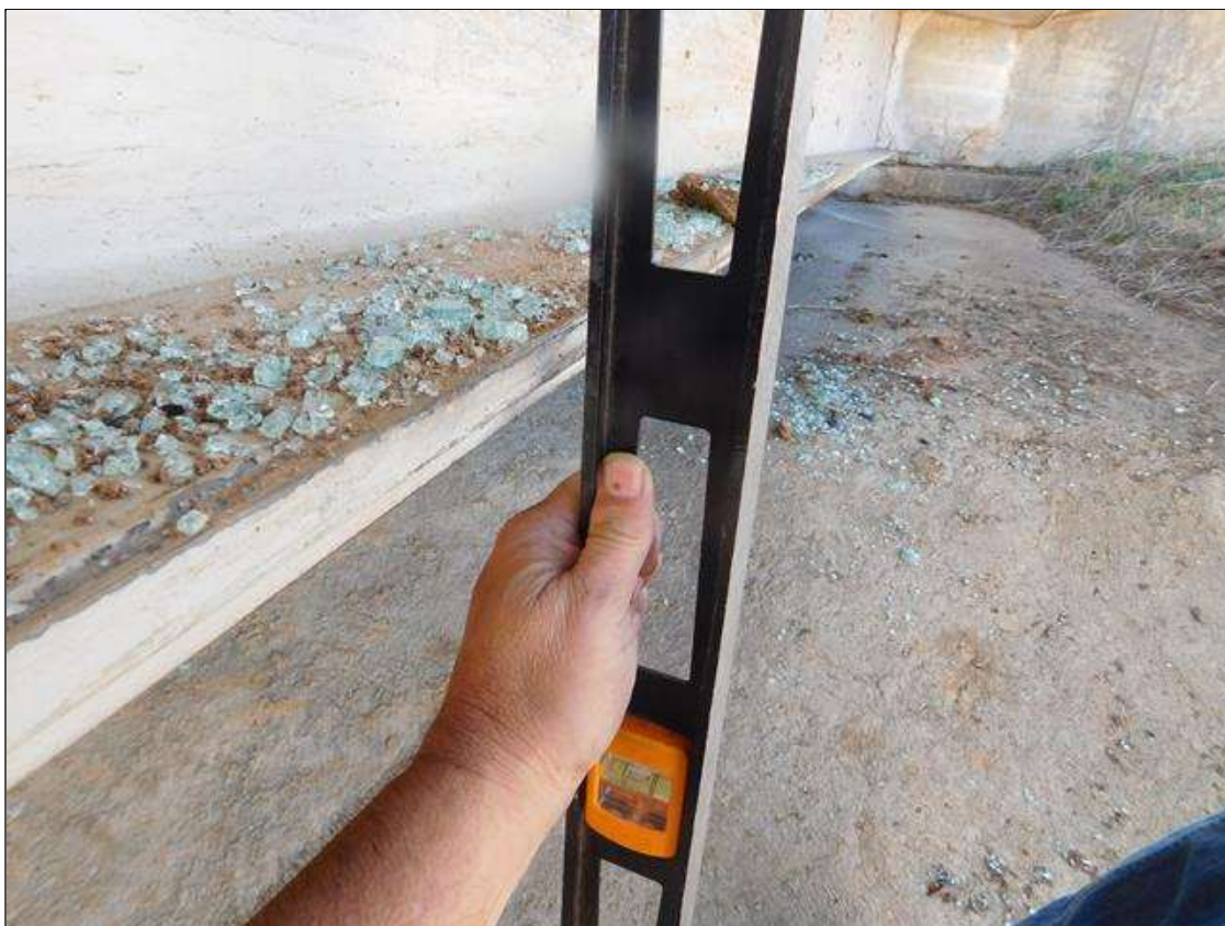
Span 1 Beam 1: IMPACT DAMAGE - THE SOUTH MOST 30' DEFLECTED 1" EASTWARD .
