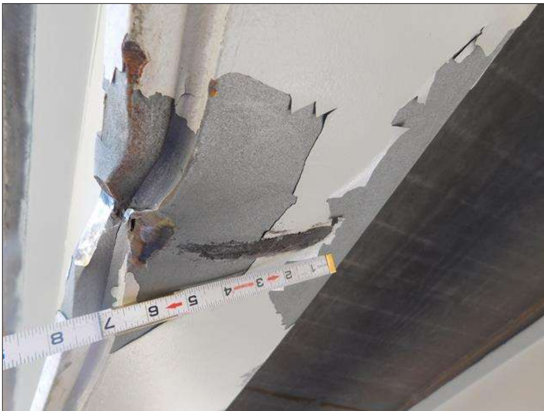
6" LONG SCRAPE ON BOTTOM OF BEAM AT POINT OF IMPACT
