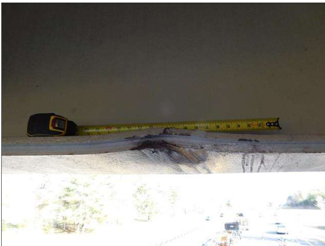
OVERVIEW OF INDENTION AT POINT OF IMPACT FOR BEAM 10. INDENTION IS 3" LONG X 1" WIDE MEASURED 26'4" FROM INTERIOR BENT 2.
