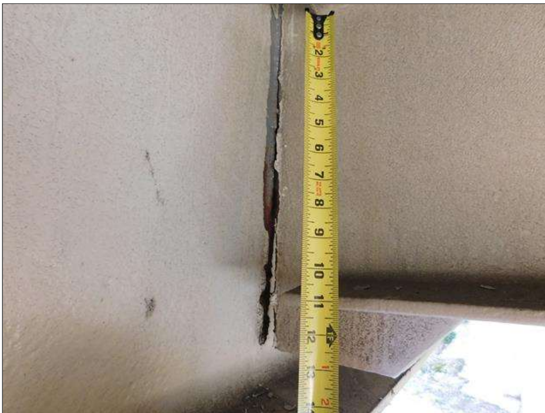
DIAPHRAGM 3 BAY 9 IN SPAN 2 IS CRACKED AND SEPERATED FROM BEAM 10. THE CRACK IS A TOTAL LENGTH OF 20" FROM THE BOTTOM OF THE DIAPHRAGM.
