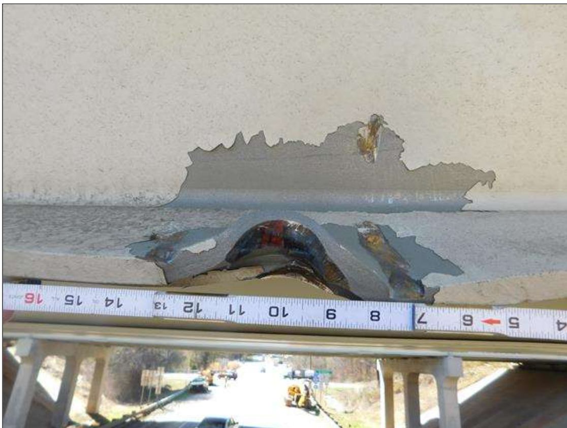
POINT OF IMPACT 1' LONG X 2" HIGH 29'-9" OUT FROM INT. BENT 1 (P/M)
