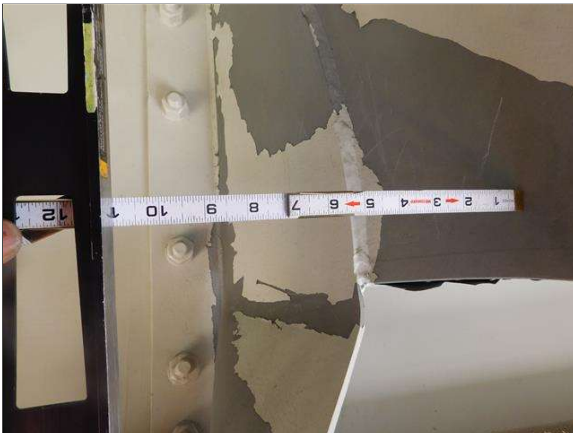
DIAPHRAGM 2 BAY 1 BENT EAST WARD FOR 11" NORTH SIDE
