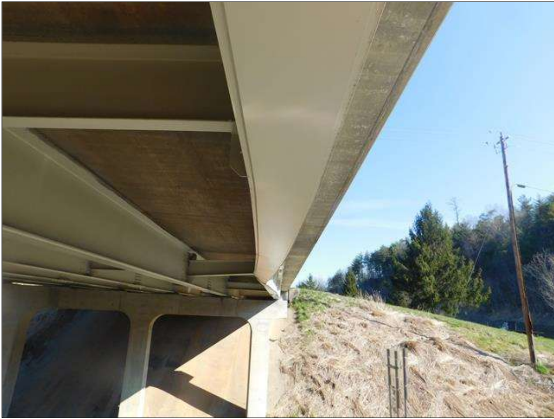
BEAM 1 SPAN 2 IMPACT DAMAGE
