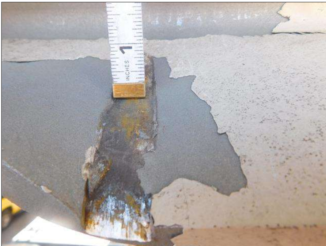
1" WIDE X4" LONG SCRAPE/ INDINTION WEST SIDE OF POINT OF IMPACT
