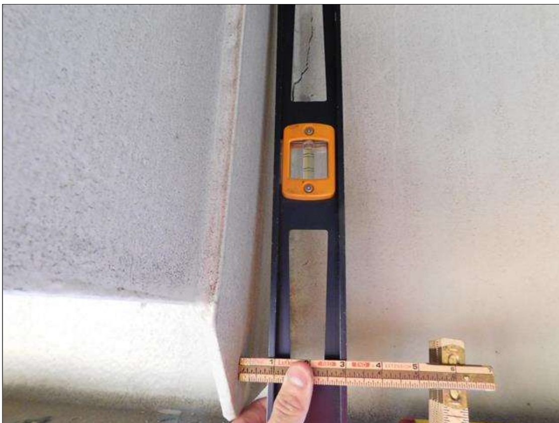
DIAPHRAGM 3 BAY 9 IS OUT OF PLUMB SOUTHWARD FOR 1"
