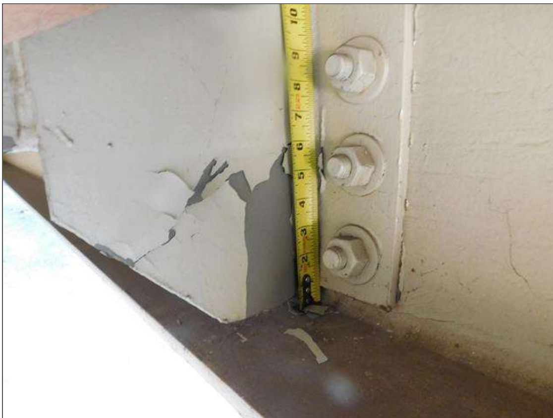
IMPACT DAMAGE - DIAPHRAGM 1 BAY 1 LEFT SIDE THE LOWER 8" OF DIAPHRAGM IS DEFLECTED NORTHWARD UP TO 2"
