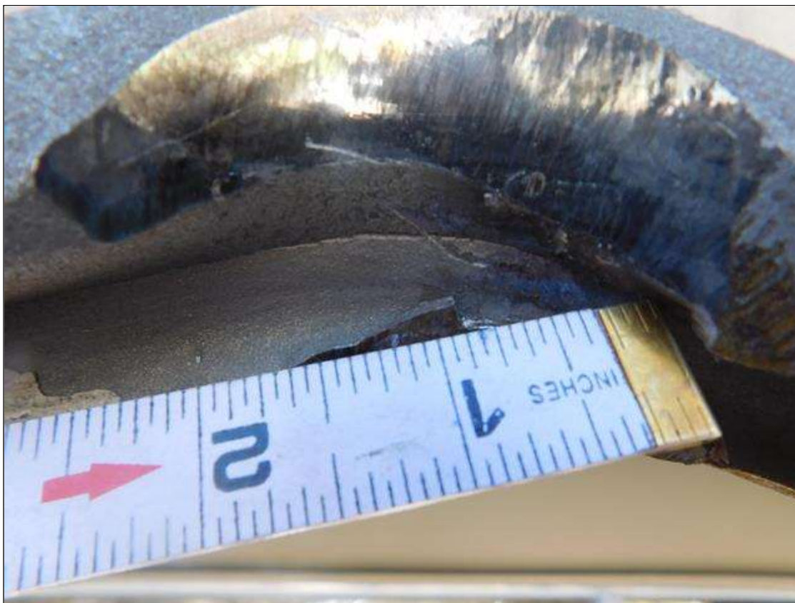
2" LONG HAIRLINE CRACK BETWEEN COVERPLATE AND BOTTOM FLANGE AT POINT OF IMPACT
