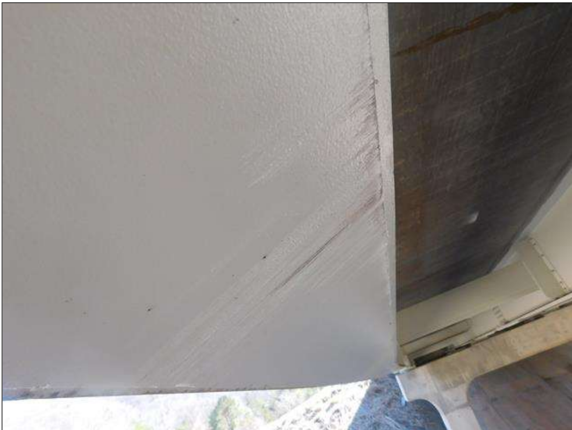
SCATTERED SCRAPES ON BOTTOM OF BEAM 1
