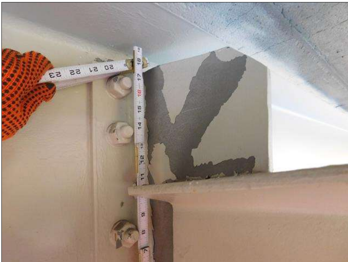
DIAPHRAGM 2 BAY 1 SOUTH SIDE BENT WESTWARD UP TO 5"
