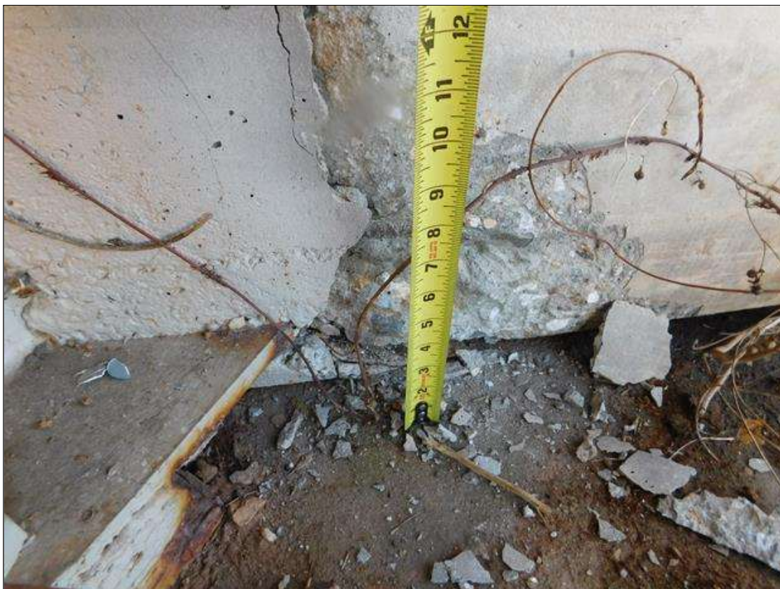
End Bent 1 Abutment/Backwall : 1'3" WIDE X 1' HIGH X 2" DEEP SPALL ON THE LEFT SIDE OF BEAM 1, WITH ONE REBAR EXPOSED .
