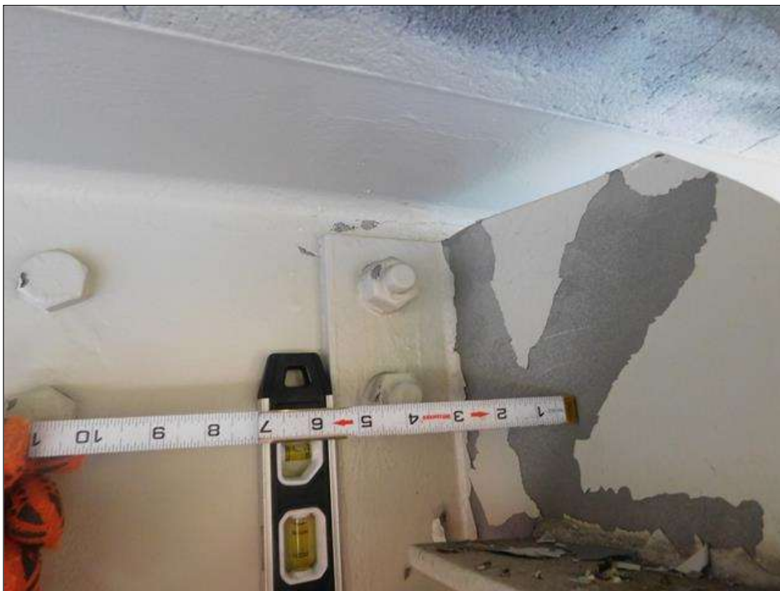
BAY 1 SPAN 2 : DIAPHRAGM 2 BAY 1 SPAN 2 IS BENT AND TWISTED WITH A 1' HIGH X 2" WIDE RIP AT ITS BASE . THERE IS ALSO A 2" LONG CRACK AT THE TOP OF THIS RIP. NORTH SIDE DIAPHRAGM 2 BENT EASTWARD 11". SOUTH SIDE IS BENT WESTWARD UP TO 5". A PRIORITY MAINTENANCE HAS BEE REQUESTED FOR THIS CONDITIONS.
