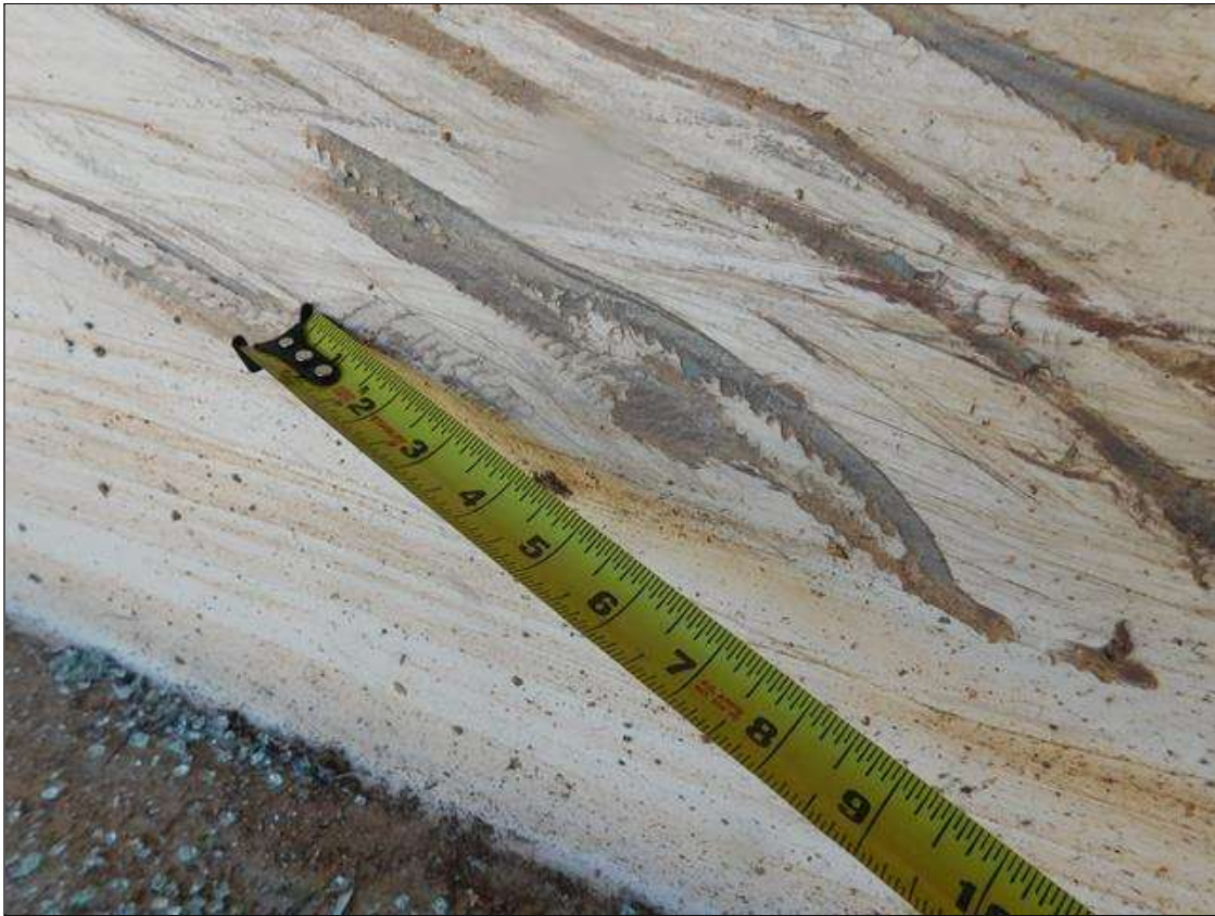
Span 1 Beam 1: IMPACT DAMAGE - THE SOUTH MOST 30' DEFLECTED 1" EASTWARD . SCATTERED SCARPES WITH 1/6" INDENTIONS THROUGH OUT A 7' LONG X 2'-7" HIGH AREA AT 12' OUT FROM END BENT 1 (POINT OF IMPACT).
