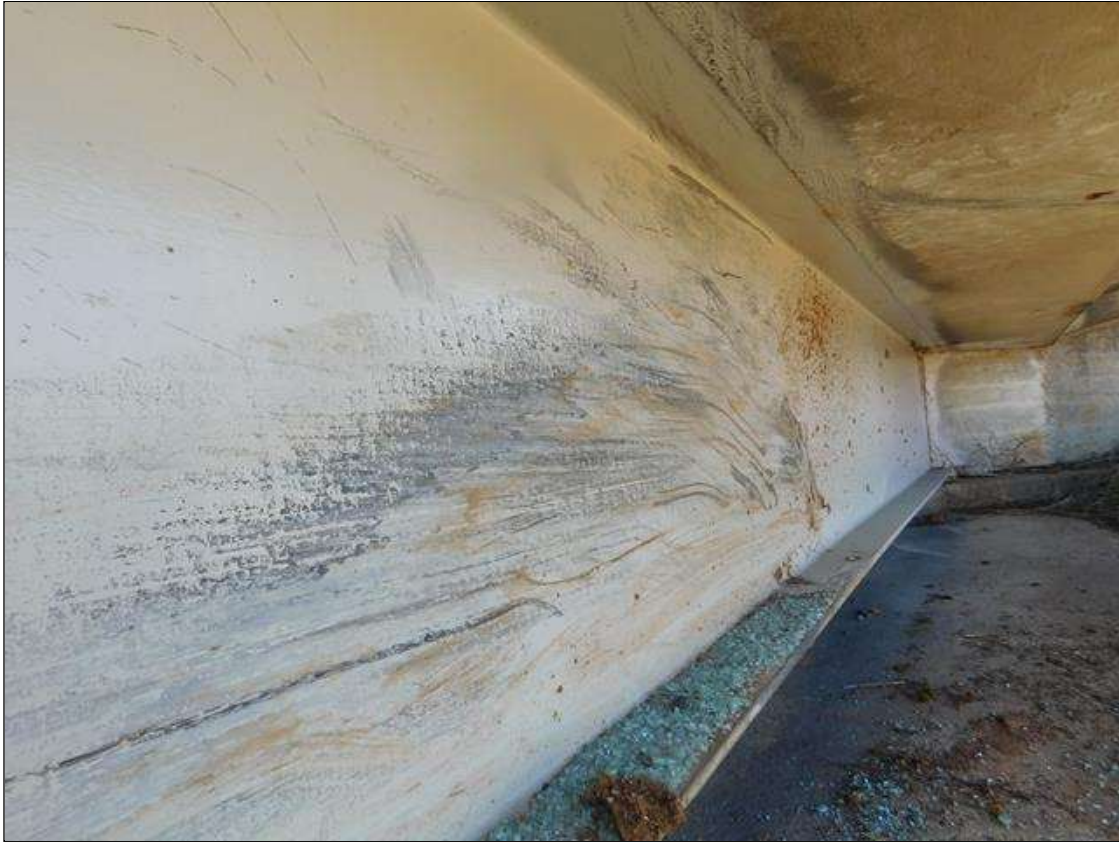
Span 1 Beam 1: IMPACT DAMAGE - THE SOUTH MOST 30' DEFLECTED 1" EASTWARD . SCATTERED SCAREPS WITH 1/6" INDENTIONS THROUGH OUT A 7' LONG X 2'-7" HIGH AREA AT 12' OUT FROM END BENT 1 (POINT OF IMPACT).
