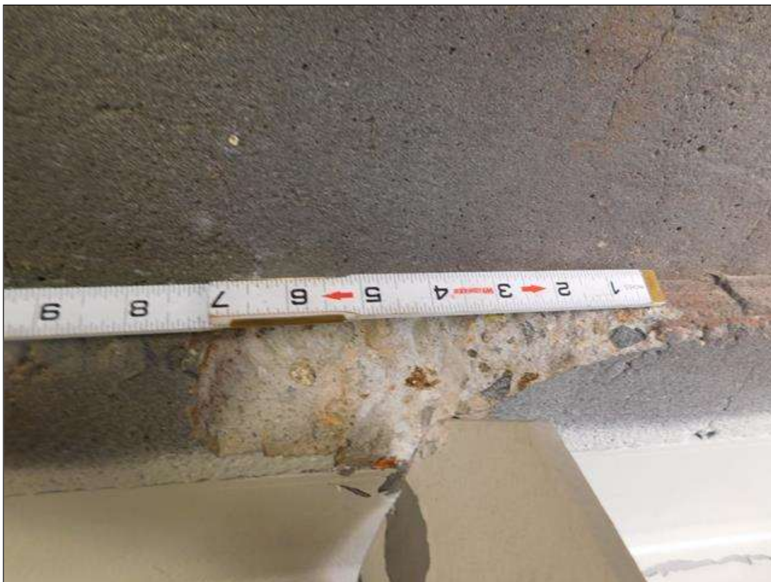
SPALLING IN BOTTOM OF DECK, 7 1/2" LONG X 1 1/2" DEEP ABOVE DIAPHRAGM 2 AT POINT OF IMPACT
