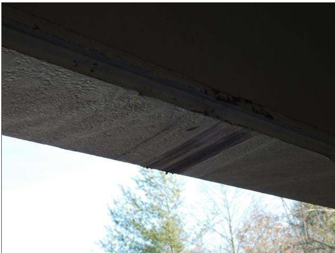
SCATTERED SCRAPES ON BOTTOM FLANGE OF BEAM 10. MEASURED 28' FROM INTERIOR BENT 2
