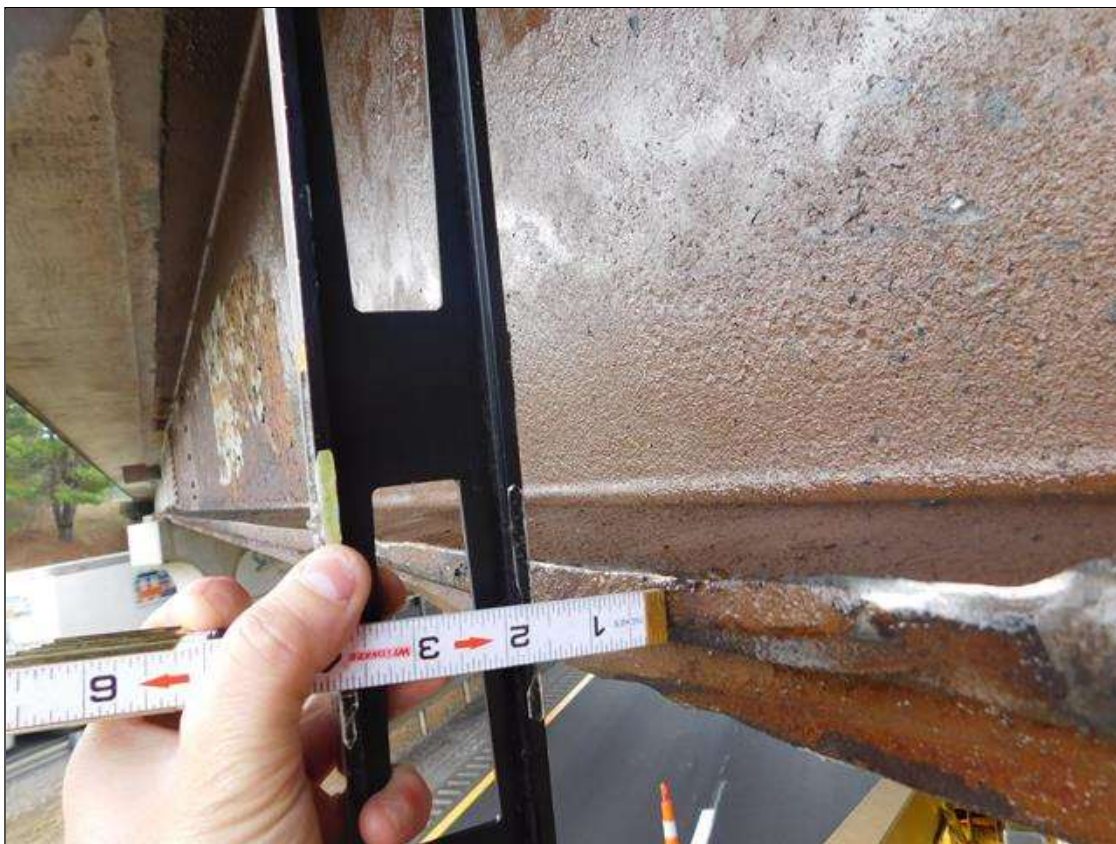
Span 3 : BEAM SWEEP EASTWARD 1.5" FOR A LENGTH OF 35' AT 29'-6" OUT FROM INTERIOR BENT 3. CONFIRMED BY SPECIAL INSPECTION ON 3/5/19
