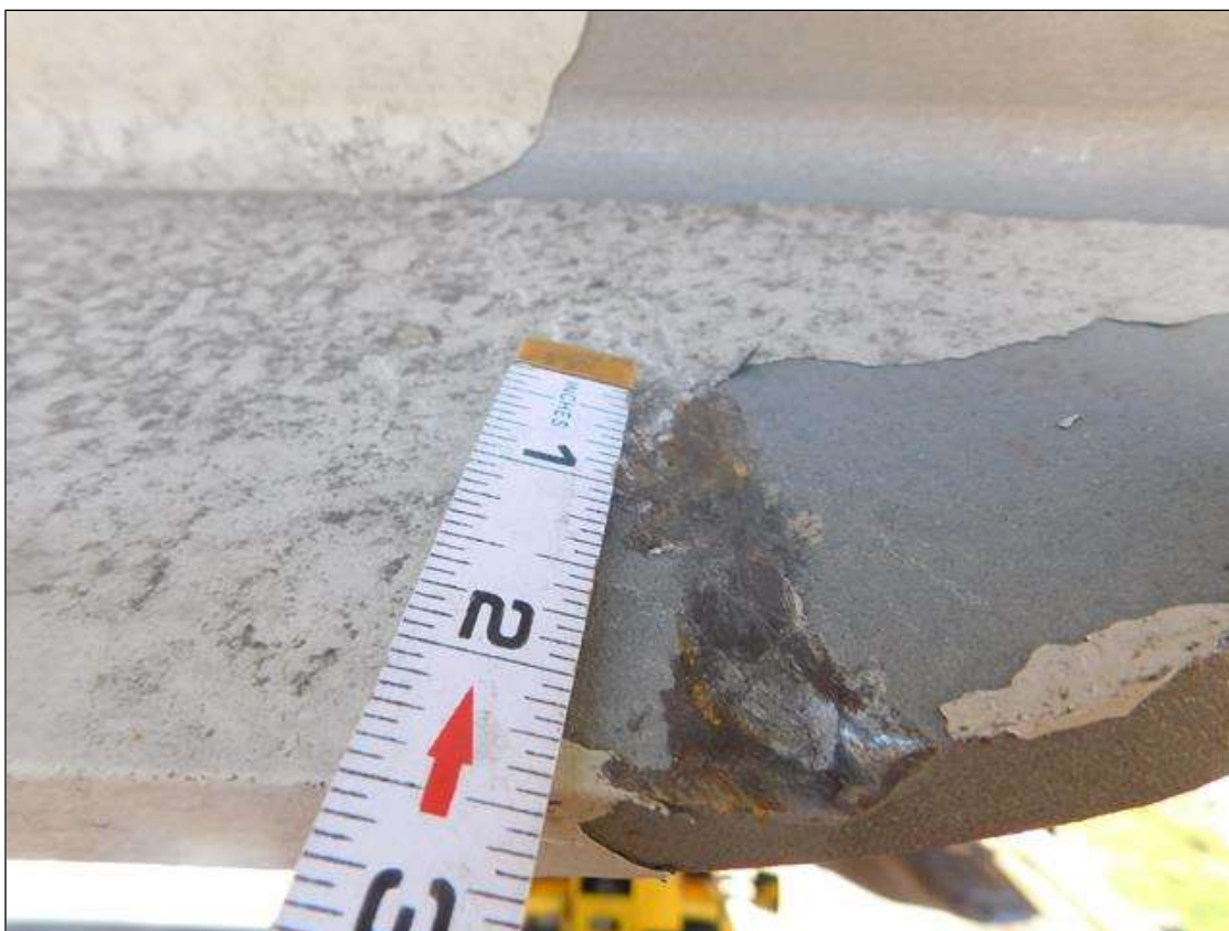
2 1/2" LONG X 3/4" WIDE SCRAPE/INDENTION EAST SIDE OF POINT OF IMPACT.
