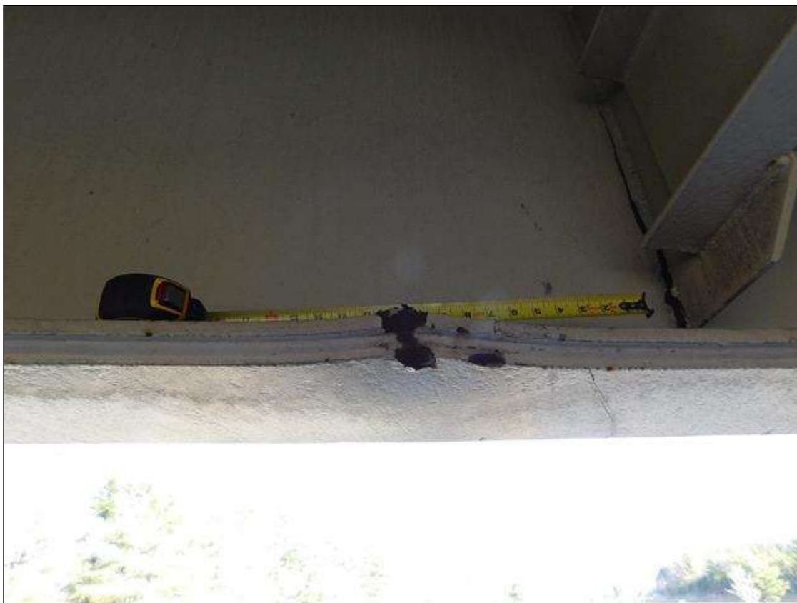
OVERVIEW OF INDENTATION AT POINT OF IMPACT FOR BEAM 10. INDENTATION IS 3" LONG X 1" WIDE MEASURED 23'2" FROM INTERIOR BENT 2
