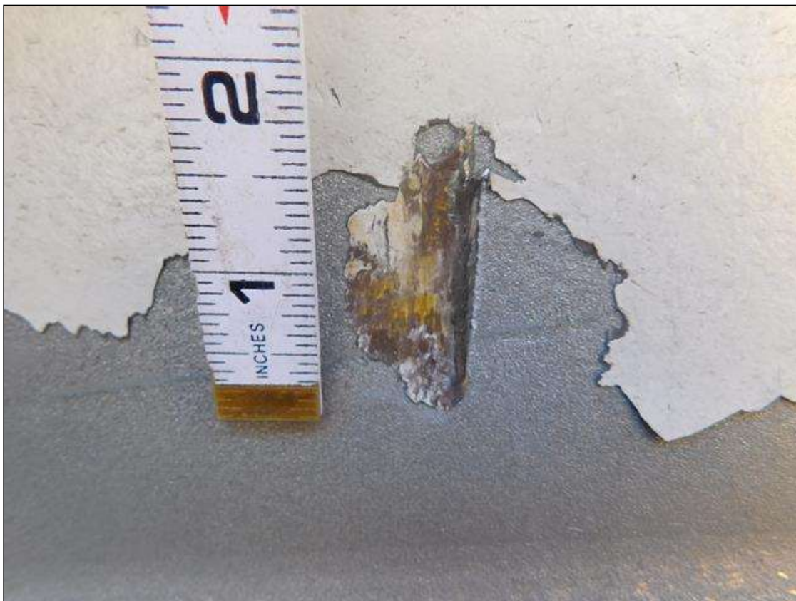
SCRAPE IN BOTTOM OF WEB 2" ABOVE POINT OF IMPACT, 2" WIDE X 1" HIGH X 1/16" DEEP
