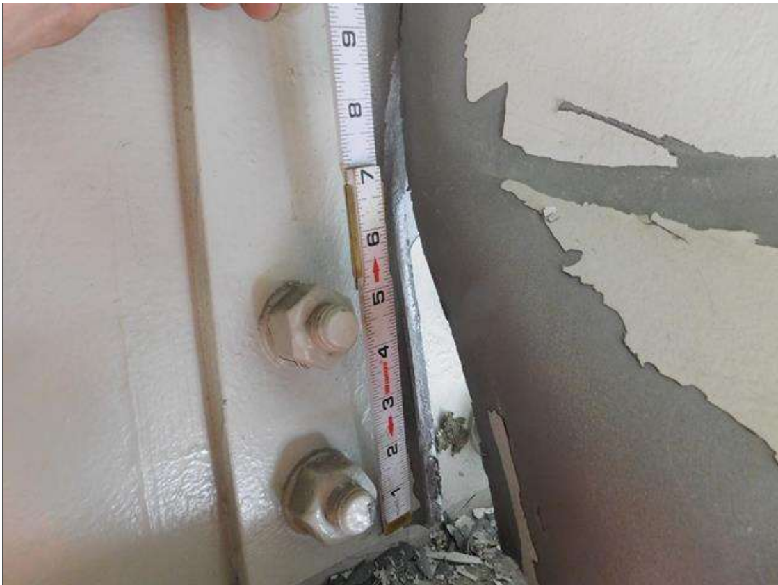
DIAPHRAGM 2 BAY 2 BENT AND TWISTED EAST WARD ON THE NORTH SIDE WITH A 1' HIGH X 2" WIDE RIP IN BOTTOM 1"
