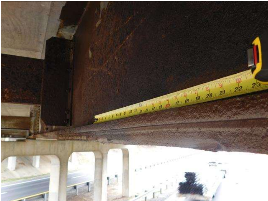
Span 3 : PREVIOUS IMPACT DAMAGE TO BEAM 5 AT 49.833' FROM IB 3, 2' LONG BY 1/2" HIGH BY 1" DEEP. CONFIRMED BY SPECIAL INSPECTION ON 3/5/19
