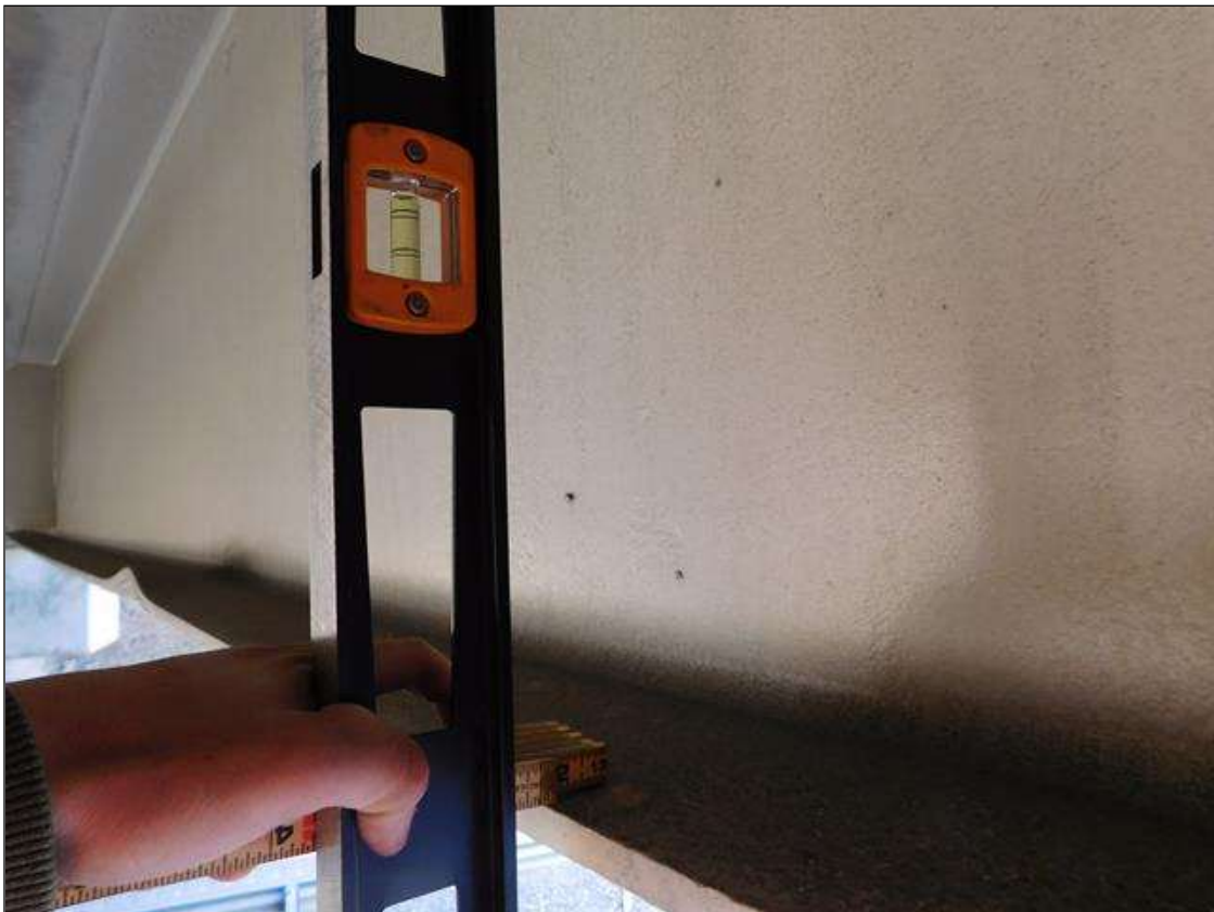
BEAM 10 IS OUT OF PLUMB WESTWARD FOR 1" FOR A TOTAL LENGTH OF 20 FEET
