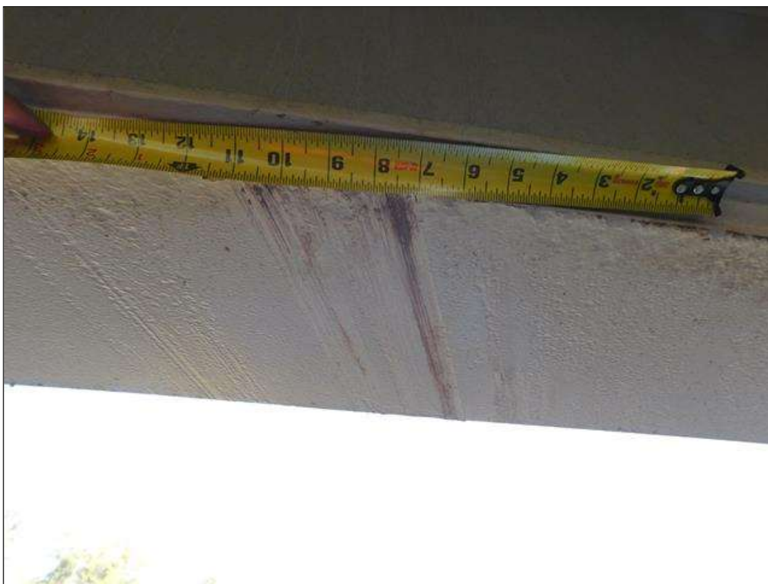
SCRAPES ON BOTTOM FLANGE OF BEAM 10 FOR A TOTAL LENGTH OF 6". MEASURED 20' OUT FROM INTERIOR BENT 2
