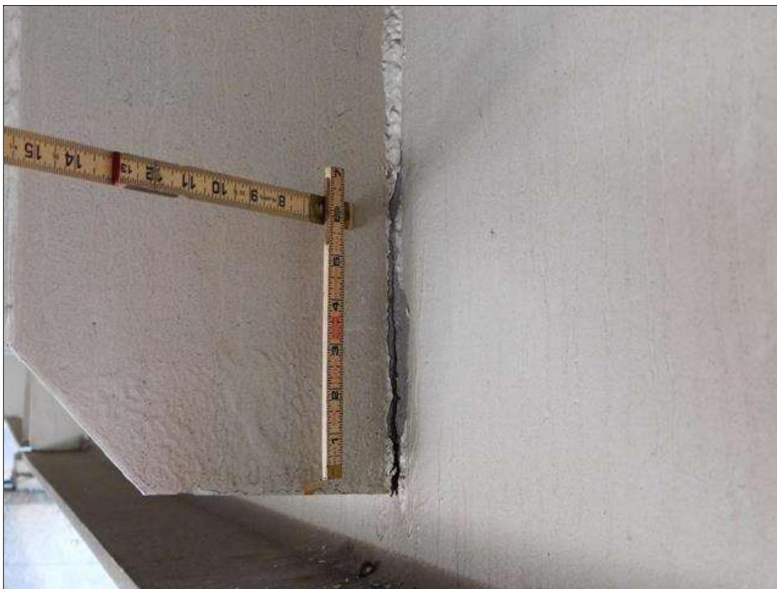
DIAPHRAGM 4 BAY 9 IN SPAN 2 IS CRACKED AND SEPERATED FROM BEAM 10. THE CRACK IS A TOTAL LENGTH OF 8" FROM THE BOTTOM OF THE DIAPHRAGM.
