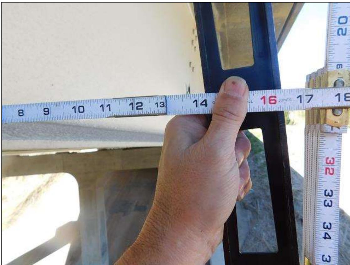
BEAM 1 DEFLECTED 1'-2" SOUTH WARD
