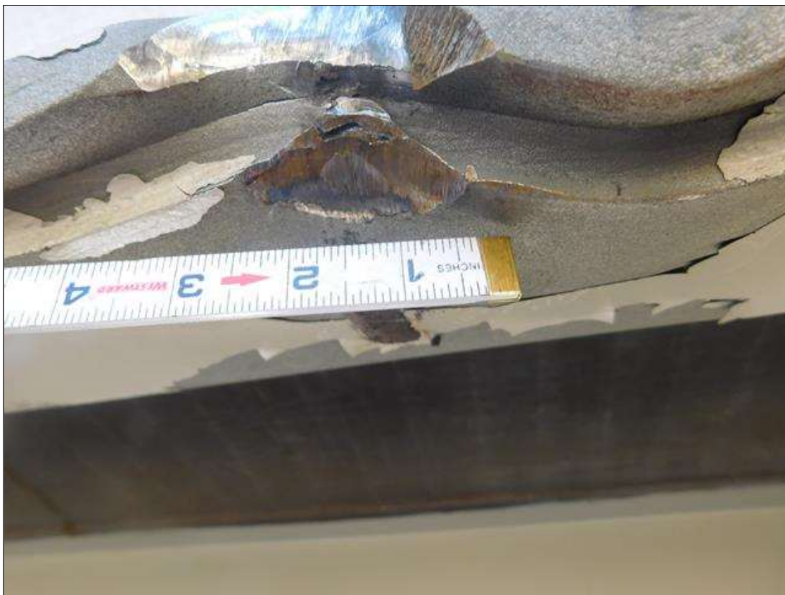
2" WIDE X 1/2" DEEP X 1" LONG INDINTION IN THE BOTTOM COVERPALE AT POINT OF IMPACT.
