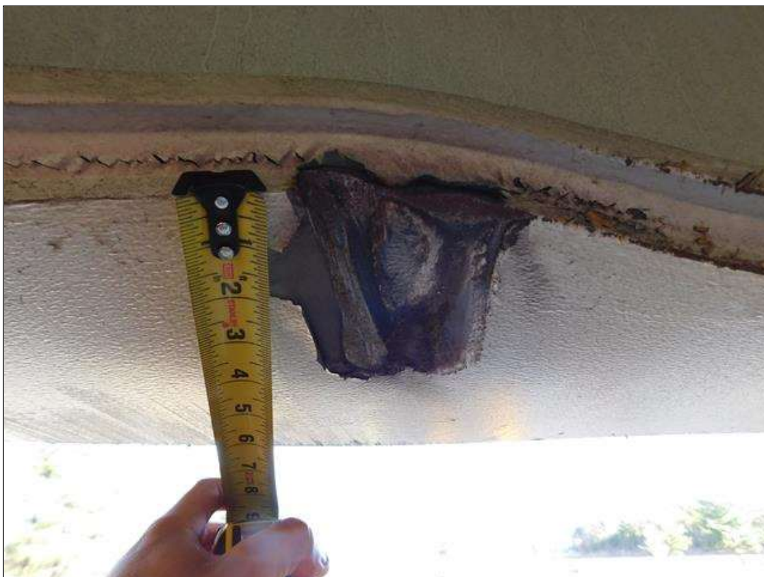
CLOSE UP OF INDENTATION AT POINT OF IMPACT FOR BEAM 10. INDENTATION IS 4" LONG X 5" WIDE IN BEAM 10 MEASURED 17' FROM INTERIOR BENT 2
