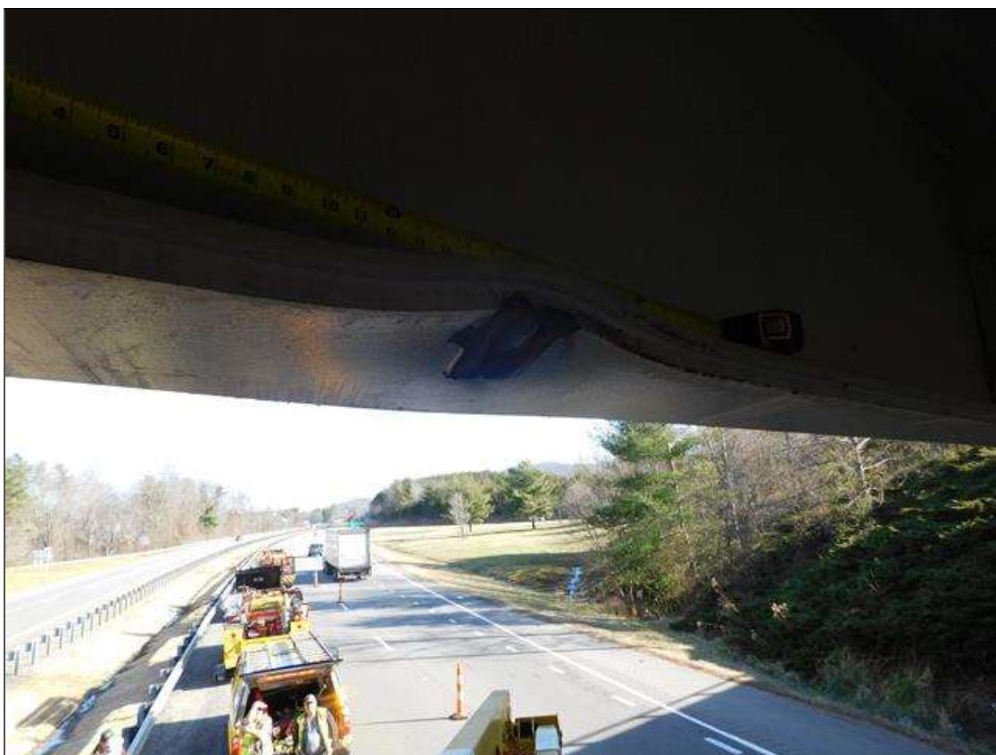
OVERVIEW OF INDENTATION AT POINT OF IMPACT FOR BEAM 10. INDENTATION IS 4" LONG X 5" WIDE IN BEAM 10 MEASURED 17' FROM INTERIOR BENT 2
