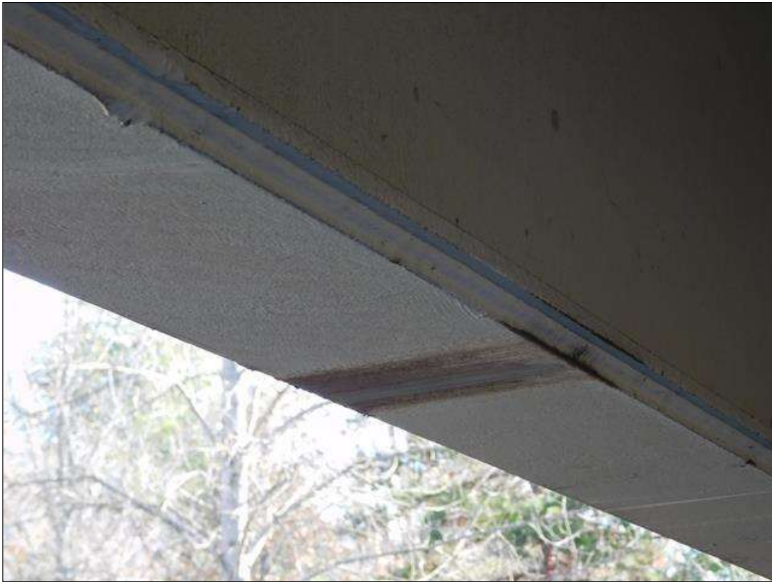
SCATTERED SCRAPES ON BOTTOM FLANGE OF BEAM 10. MEASURED 30' FROM INTERIOR BENT 2
