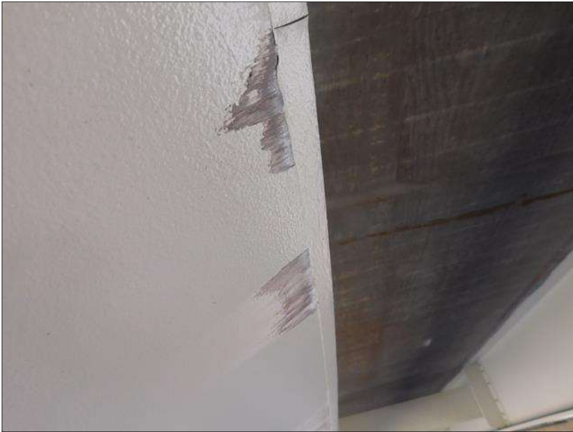
SCATTERED SCRAPES ON BOTTOM OF BEAM 1
