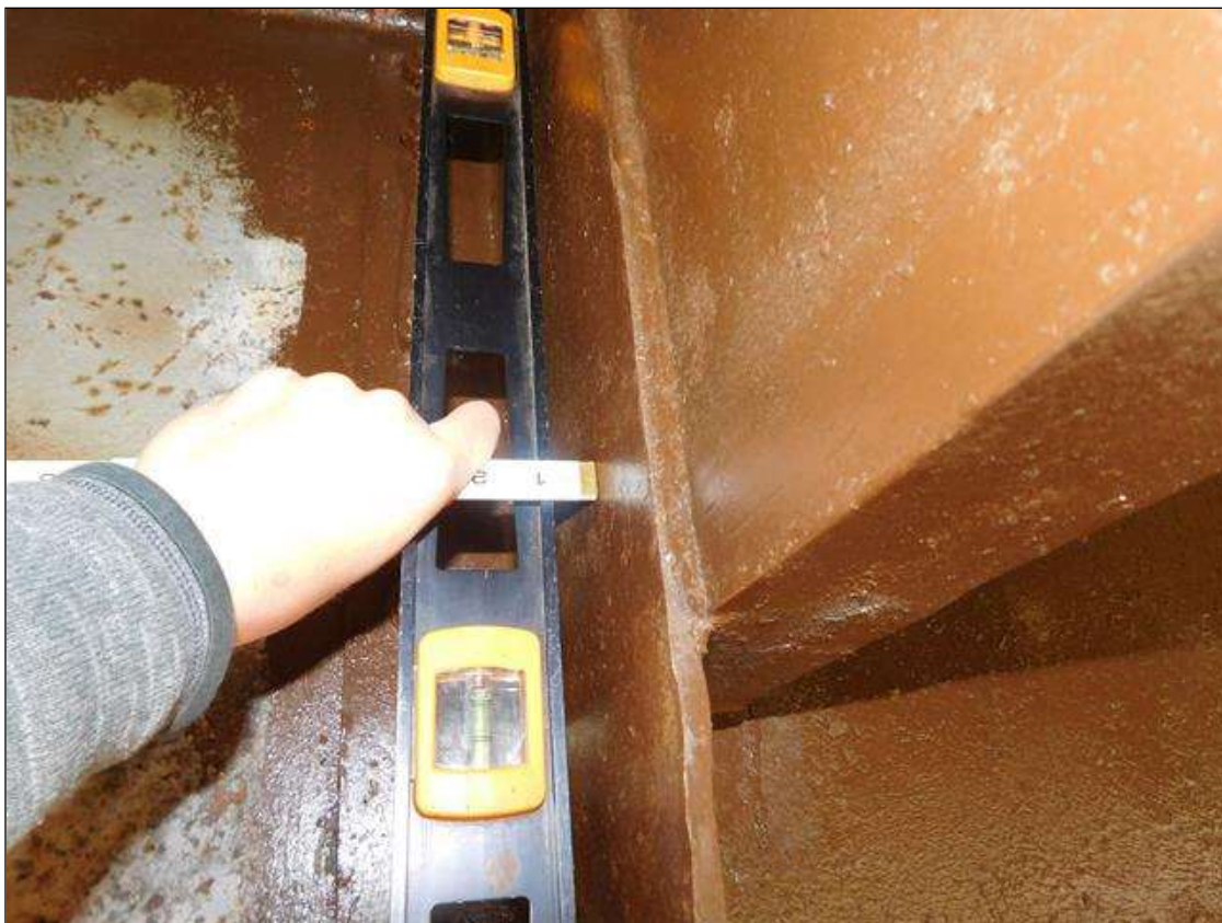
PREVIOUS IMPACT DAMAGE TO DIAPHRAGM 4 BAY 5. SWPET NORTHWARD 1/2"
